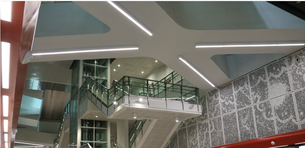
Singapore MRT Station - Thomson-East Coast Line
